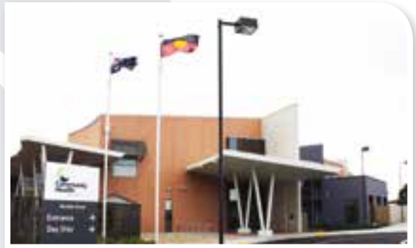
Morwell 81-87 Buckley Street
