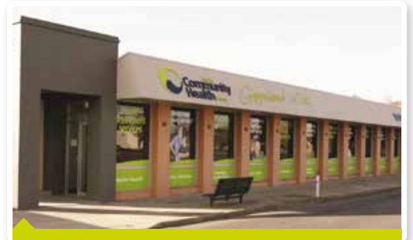
Traralgon Corner Princes Highway and Seymour Street
