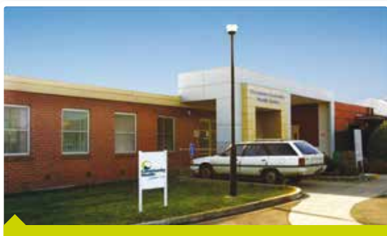
Korumburra Gordon Street, at Gippsland Southern Health Service
